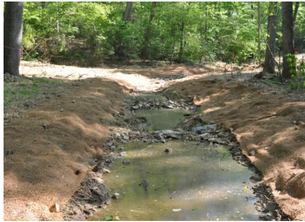
Photograph 4: View of new channel facing downstream
