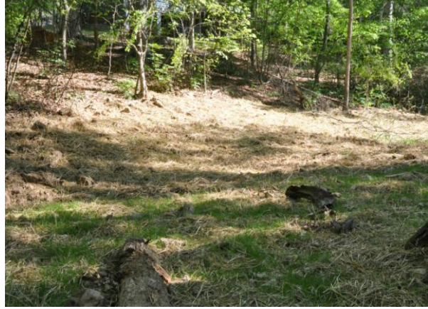
Photograph 2: Old channel filled in and eroding hillslope stabilized
