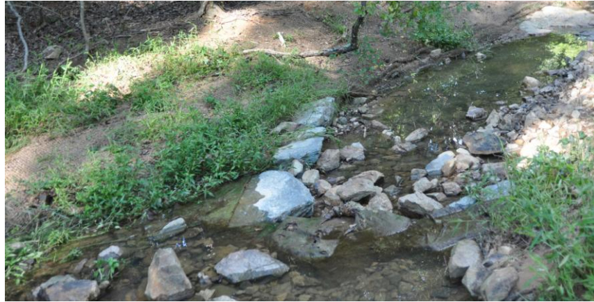
Photograph 6: J-hook boulder structure
