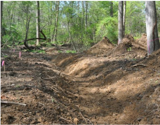
Photograph 3: New channel constructed
