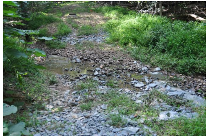
Photograph 9: Stabilized sewer easement crossing
