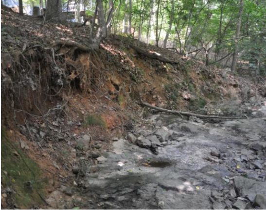
Photograph 1. Eroding hillslope before construction.
