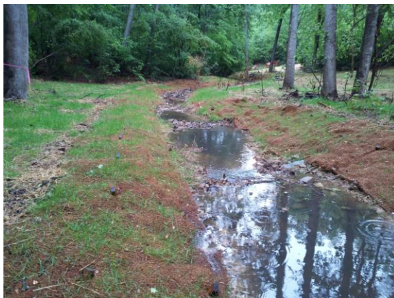
Photograph 5: View of matting after a bankfull event a few weeks after construction
