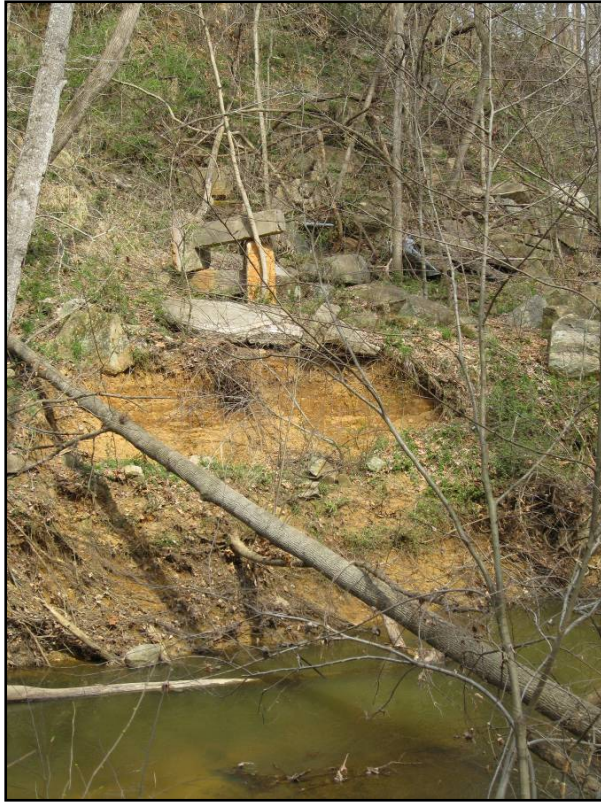
Construction debris from past highway widening on the steep slopes below Hwy 54. This is the north streambank of Morgan Creek.
