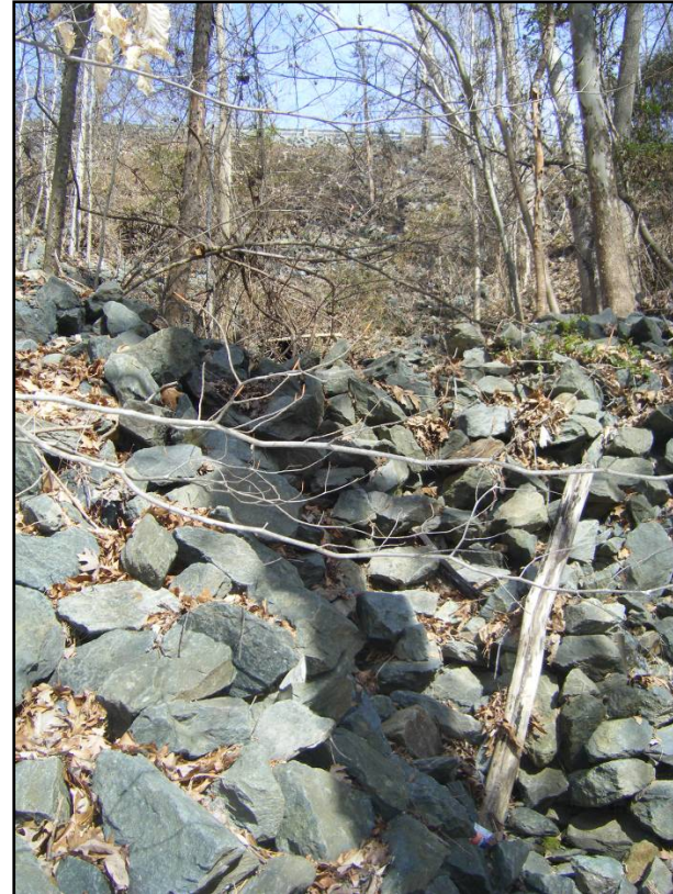
Rip-rap storm drainageways from Hwy 54 (guardrail on the highway is visible at the top of the photo).
