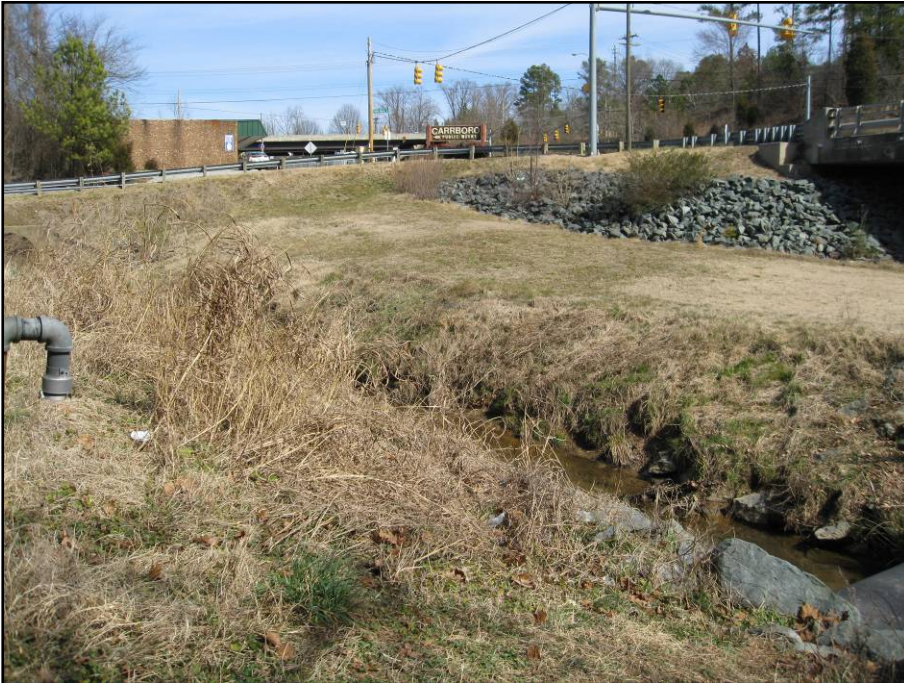
Driveway access to the Town property and drainageway in front of the Town of Carrboro Public Works site near the Smith Level Road bridge.
