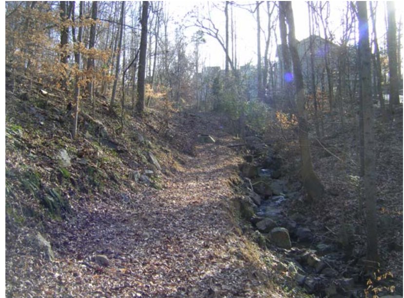
Steep stretch of OWASA easement approaching Villages of Chapel Hill driveway.
