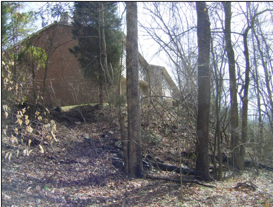
Canterbury Townhouse Property, north side of the creek.
