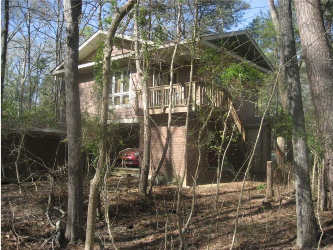
Secondary Dwelling / Garage at 300 James Street
